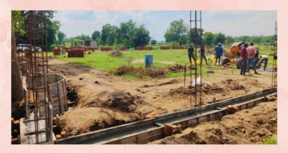
started phase-I construction of 1650 feet long and 7 feet high boundary wall
